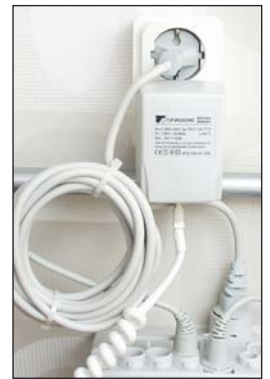
The picture shows a double wall socket, to which the control unit as well as the transformer for the lighting are connected.
